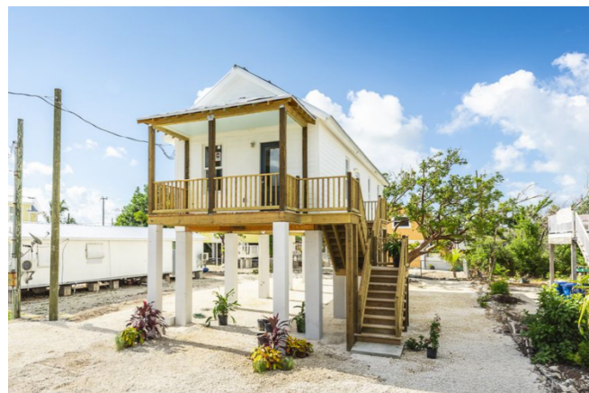
One of the first four homes to be completed by FKCLT. This site was purchased by a resident eager to leave after the storm. The new homes are raised to protect from future flooding and built to resist windspeeds of 200 mph. Credit: FKCLT
