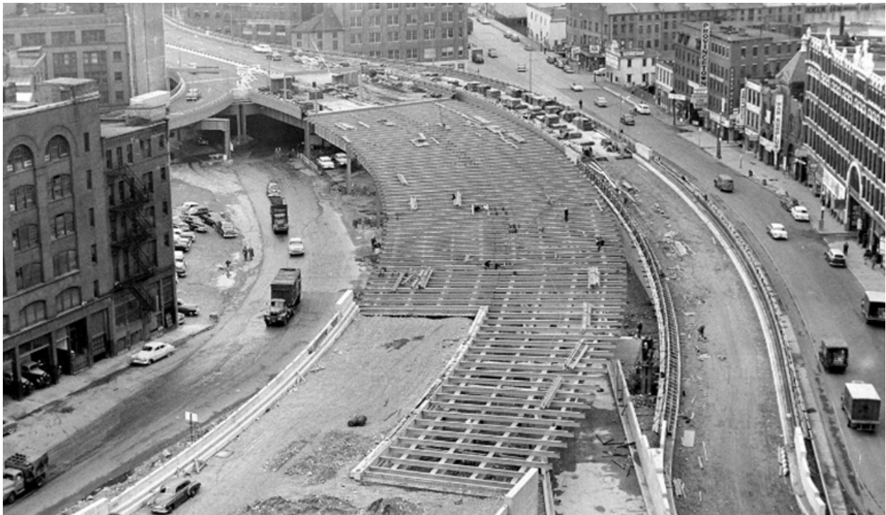
Figure 7 Construction of central artery 1954
