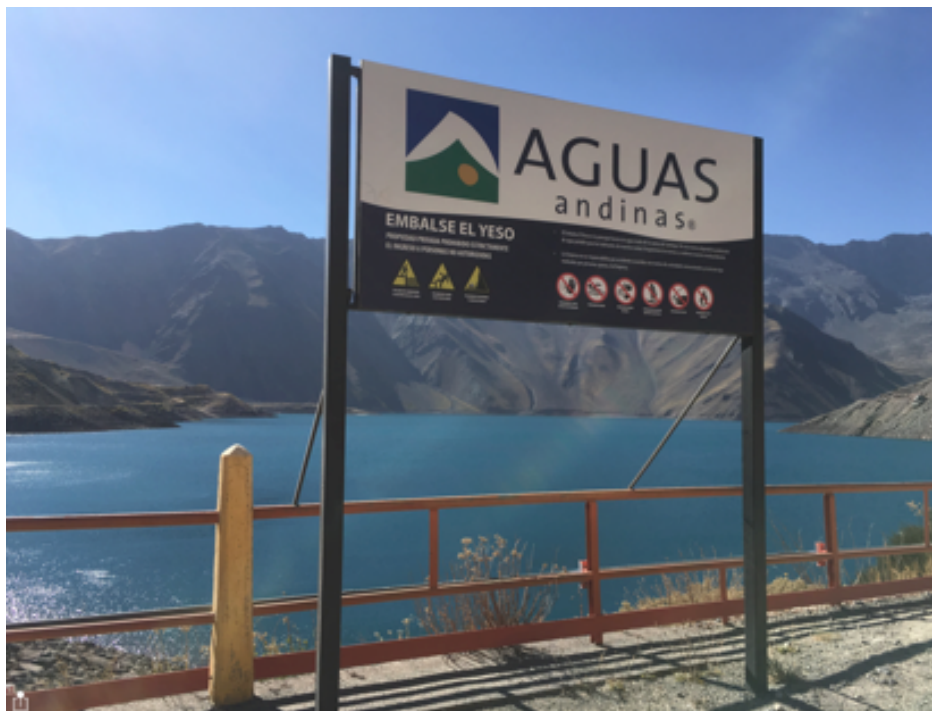
Figure 7: El Yeso Dam, high in the mountainous upper catchment of the Maipo River, owned and managed by Aguas Andinas (Photo by Author, May 2018).
