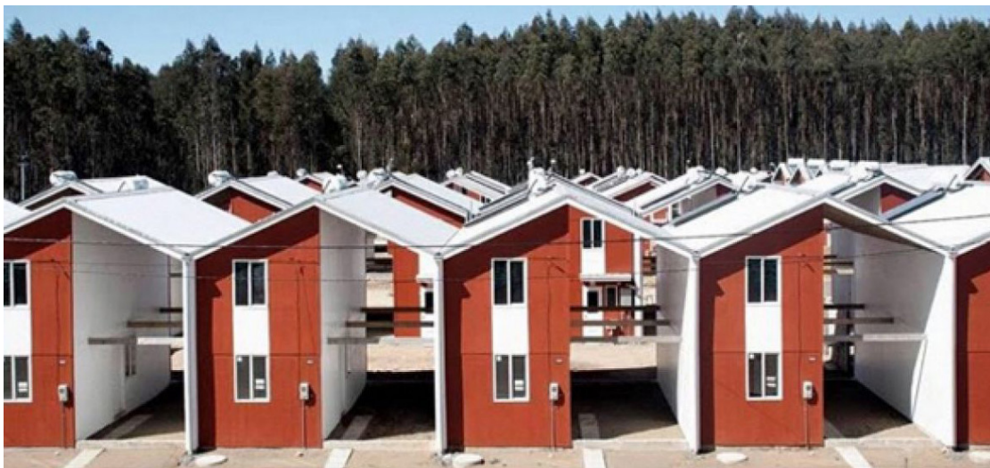
Villa Verde, completed in 2016, is one of Elemental's most recent iterations of the "half a house" concept. Source: El Contrista
