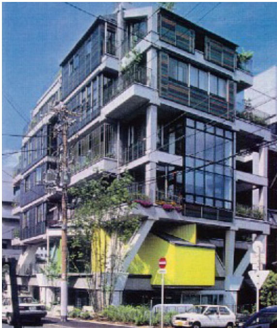
Next 21 in Osaka was one of the first built examples of John Habraken's open building concept. Source: habraken.com
