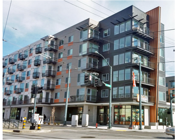
Five-over-one construction is cost effective but typically has bland and rigid aesthetic qualities. Source: nishkian.com
