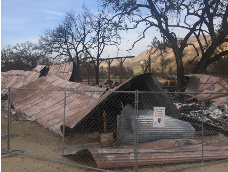
Figure 12 – Paramount Ranch Old Western Town, fire damage
