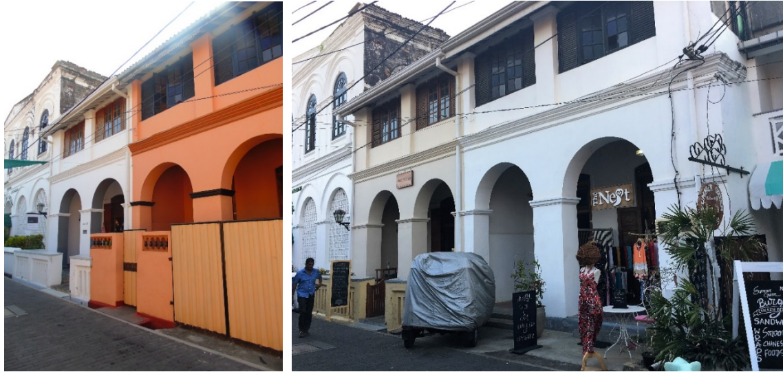
Figure 4.10. Church Street modern additions of gates and walls removed, and façade repainted white. The property has been converted to commercial uses, Sources: (Left) Image from GHF dated 2014; (Right) Photo by author in 2019.
