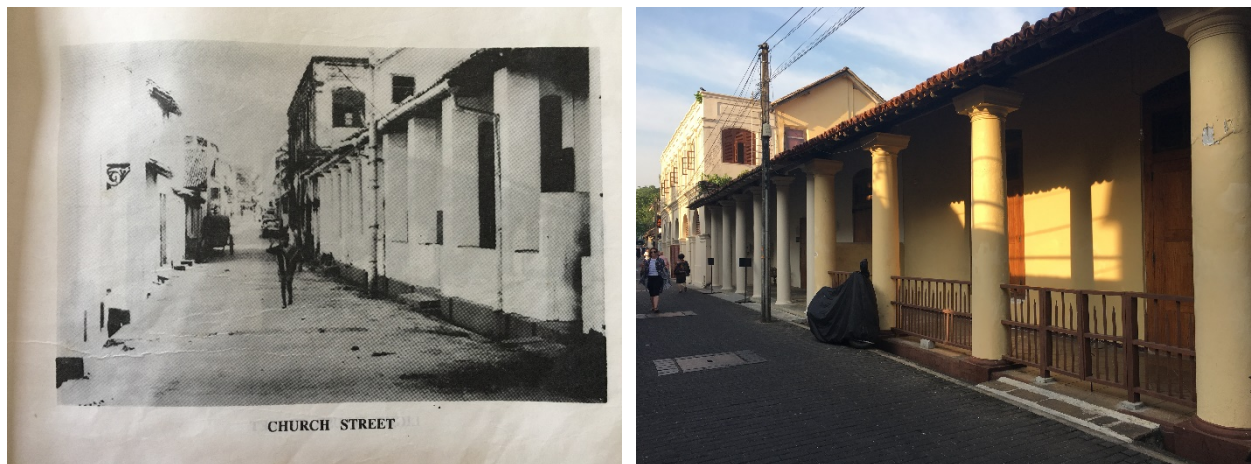
Figure 4.6. Church Street restoration of façade architectural elements to original Dutch form, Sources: (Left) Image from “The Conservation of the Galle Fort and its Environs” (Kuruppu and Wijesuriya 1992) dated 1990; (Right) Photo by author in 2019.
