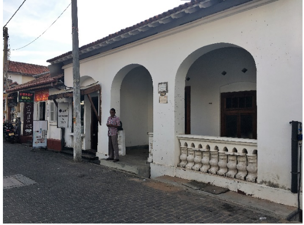
Figure 4.7. Number 72 Church Street façade conservation which involved restoring Dutch arches and removing later additions, Sources: (Left) Image from GHF dated 2007; (Right) Photo by author in 2019.
