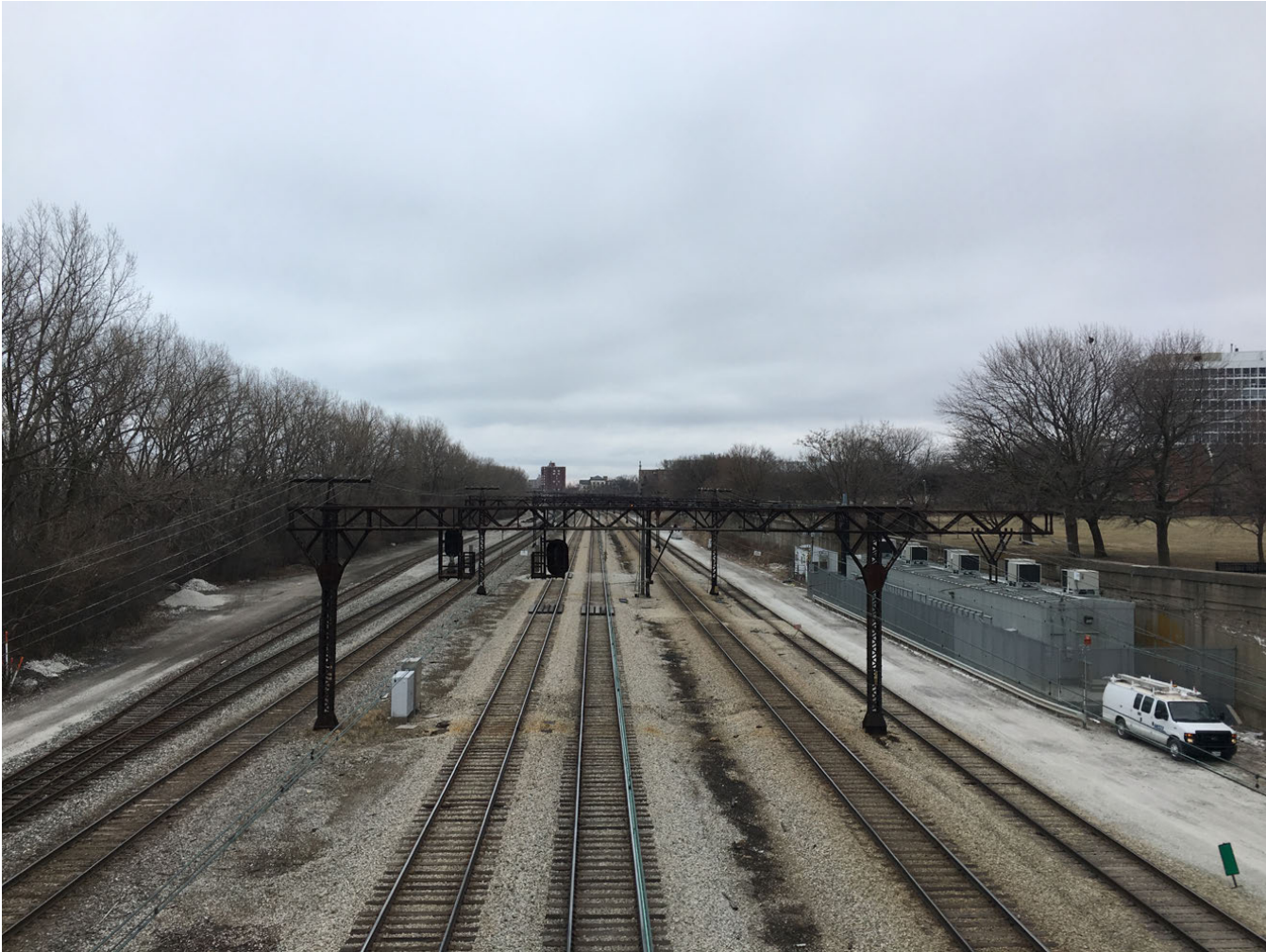
31st Street Overpass, Illinois Central Railroad
