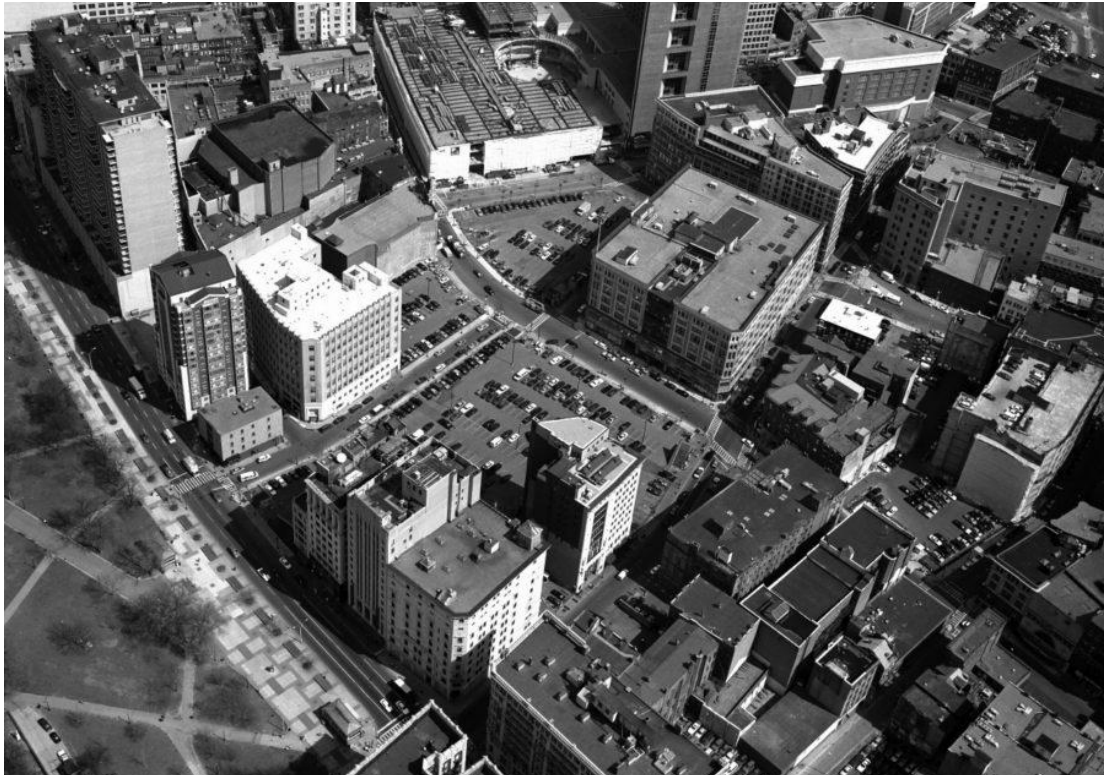
The vacant project site in 1995.
