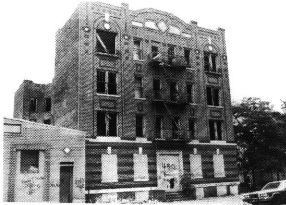
Sterling Street Housing Corporation Development Project located on Sterling St., in Brooklyn, N.Y. (19 Units)
