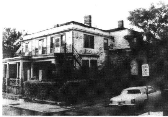
VBCDC's Single Room Occupancy Development Project located at 6 Hartford St., in Roxbury (18 SRO's)
