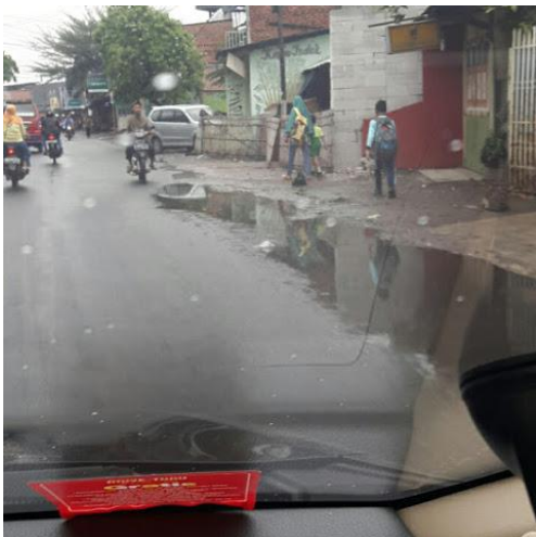
(c) Stagnant water on the road
