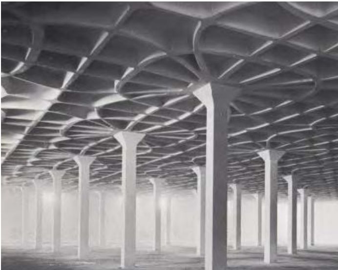
Figure 6 Stress-line-inspired architectural precedents: Above: Gatti Wool Factory floor system (Halpern, Billington, and Adriaenssens 2013) Below: Catalano's spherical design proposal (Allen 2010)
