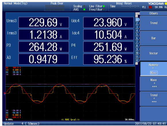
Fig. 11. Line voltage (red), line current (yellow), output voltage (blue) and output current (purple) for the following operating point: input of 230 Vac output voltage of 24 V and output power of 251 W. The power factor is 0.948 and efficiency 95.236%. This data point is taken including all the software changes that increase efficiency. The converter does not draw peak current when the voltage is maximum.
