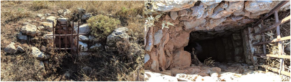
Figure 13. Small drain feature in Meteles Depression (Photos by A. Koh)
