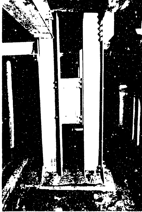
Figure 2.4 Zinc plating line substructure, Johnstown.
