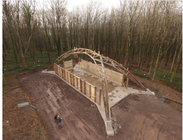
Figure 9. Wood Chip Barn arching truss, completed (Mollica and Self 2016, 140)
