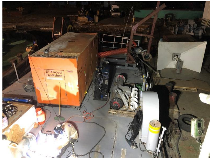
FIG 80 The team worked past midnight on November 18 th to finish welding work and fix a constraint issue with the co-axial auger (notice co-axial device removed; discussed more later on). The team was accustomed to working down to dusk, but power usually shut off around 5:00pm. This night, the team rented a generator to run the aluminum welding machine. Also pictured is a local welder sealing a hatch that had been cut to remove the engine for repairs at one time.
