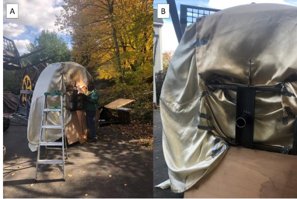
FIG 71 The lay-flat hose storage reel had plates and a central tube added to it such that it could be easily transferred to the pilot hose reel once in the DR. Credit to Bob Gray for this idea. (A) Brendan Newton welding channel onto the side of the lay-flat hose storage reel. (B) Close-up of welded channel and central 3.5" tube turning freely inside. The layflat hose was protected from spatter by a welding blanket.
