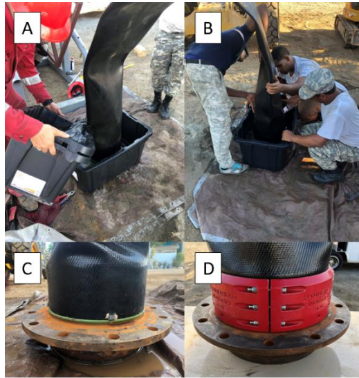
FIG 88 (A) Folkers Rojas pouring boiling water around the custom fitting in an attempt to stretch the end of the layflat hose, using the thermal expansion of the metal fitting, such that there might be more clearance when the system came back to equilibrium, (B) the GC-111 crew applying brute force to try to coax the layflat hose onto the custom fitting, (C) the custom fitting completely installed in the end of the layflat hose, (D) the groove-loc collar securing the custom fitting inside the layflat hose.
