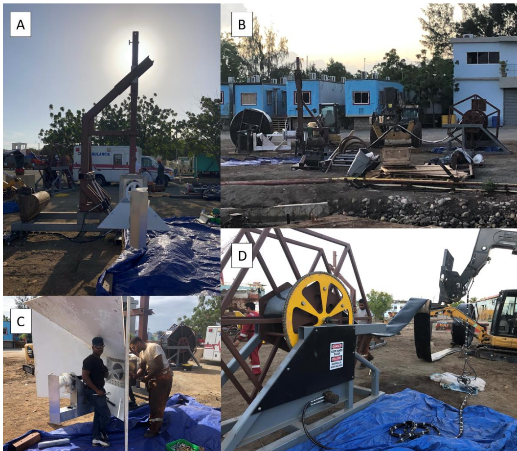
FIG 70 (A) crane and coaxial inlet being assembled in staging area. (B) the staging area in which the layflat hose can be seen getting transferred from the storage reel onto the pilot hose reel. (C) The GC-111 crew finishing tightening all 400+ bolts in the coaxial inlet funnel. (D) Close-up of the layflat hose being transferred onto the pilot hose reel. The storage reel spins freely on two steel sawhorses. The telehandler supports/tensions the hose while also providing hydraulic power to the pilot hose reel.
