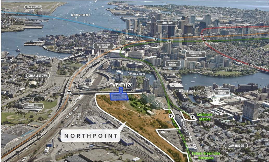
Figure 2. North Point at the Intersection of Three Cities, Source: HYM Investment Group.
