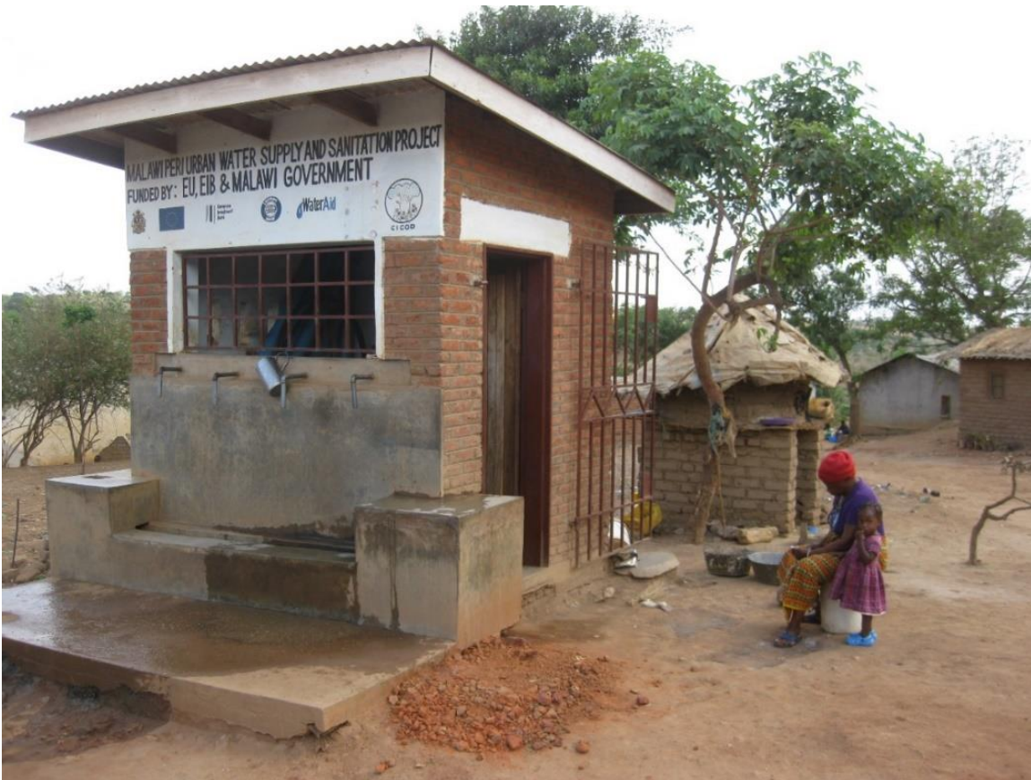
Figure 5.7. Water Kiosk in a Peri-Urban Area of Lilongwe, with Kiosk Attendant
