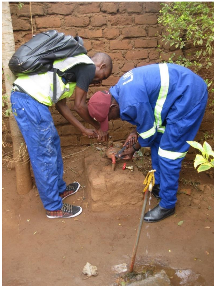
Figure 5.12. Team of Plumbers Replacing a Stuck Water Meter, Southern Zone
