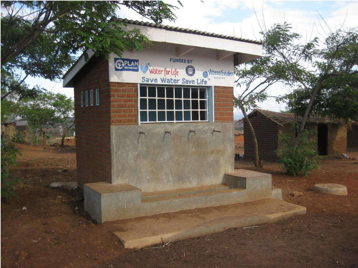
Figure 5.8. Water Kiosk in a Peri-Urban Area of Lilongwe, Newly Constructed
