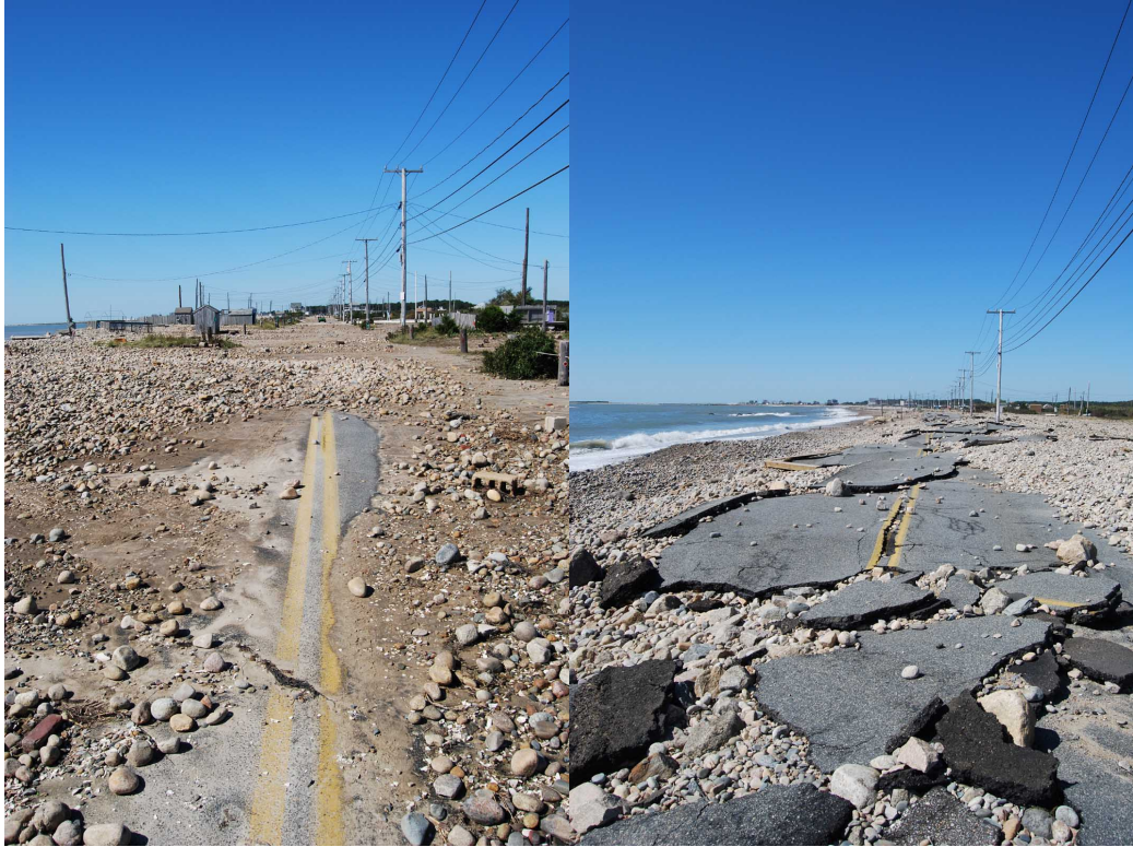
Figure 10: Two images of East Beach road after it was overwhelmed by flooding during Hurricane Irene in 2011. Source: https://buzzardsbay.org/enjoy-buzzards-bay/weather/storms-hurricanes/tropical-storm-irene-buzzards-bay/ .
