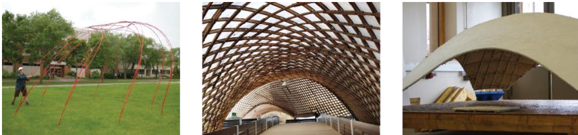
Figure 3.1: Three examples of bending active structures. From left to right: bending-active frame, bending-active gridshell with a flexible membrane, and hybrid bending-active gridshell integrating a rigid shell. Central picture © Hubert Berberich (CC-BY 3.0).
