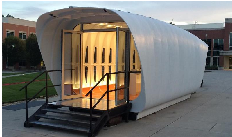
Figure 1-9: 3D printed home designed by Oak Ridge National Laboratory printed on the BAAM with fiber reinforced polymer [30].
