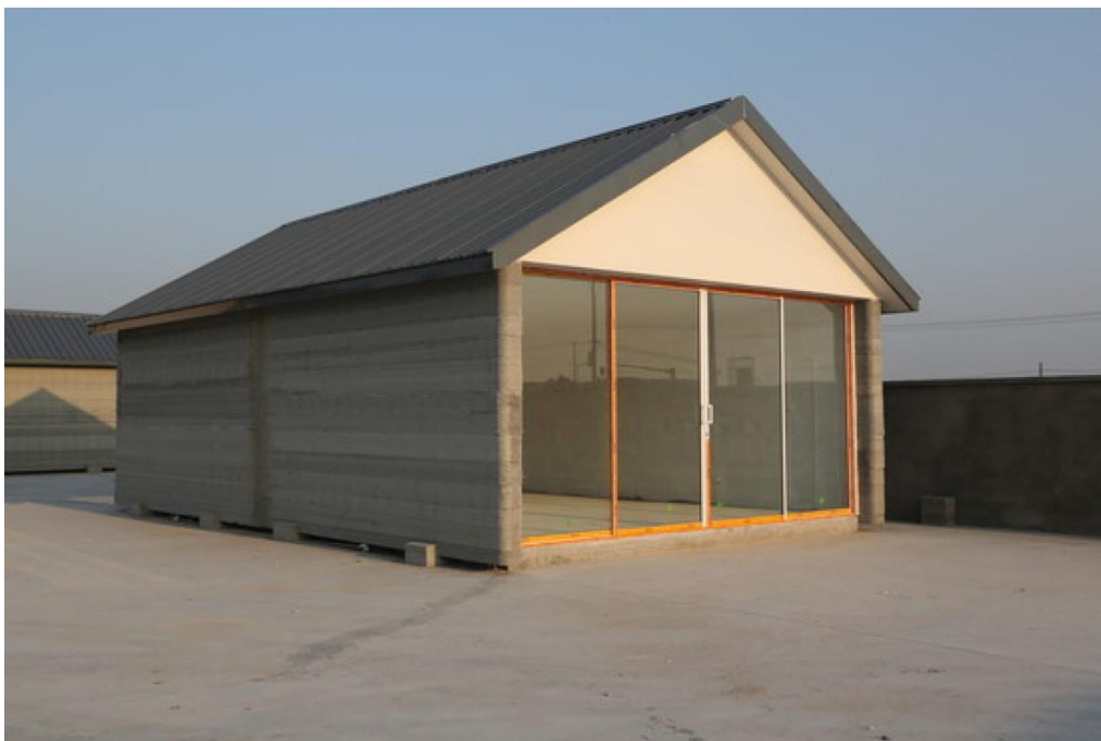
Figure 1-5: 3D printed home by Winsun that completed 10 similar homes in 24 hours printing with a glass/concrete mix. Each home was 16,500 square feet and costs less than $5000 [26].
