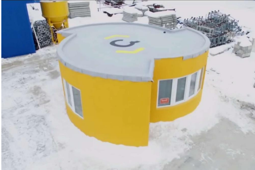
Figure 1-6: 3D printed concrete home constructed by Apis Cor in extreme elements. Printed in less than 24 hours costing ~$10,000 [24].
