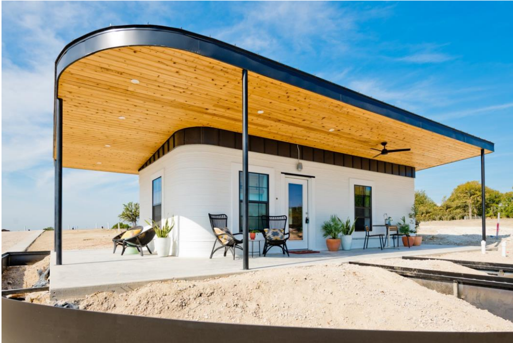
Figure 1-4: 500 square foot concrete home 3D printed in 27 hours by ICON built in Austin, Texas.[25]
