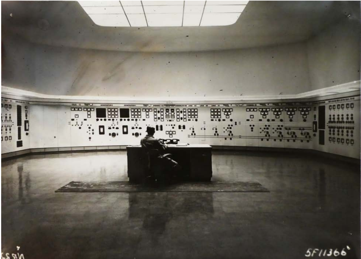
Figure 26 Unidentified control room. Photography on display in the 1949 exhibition. Unknown photographer, Fagsaker, Norske Arkitekters Landsforbund Archives, The National Archives of Norway, Oslo.
