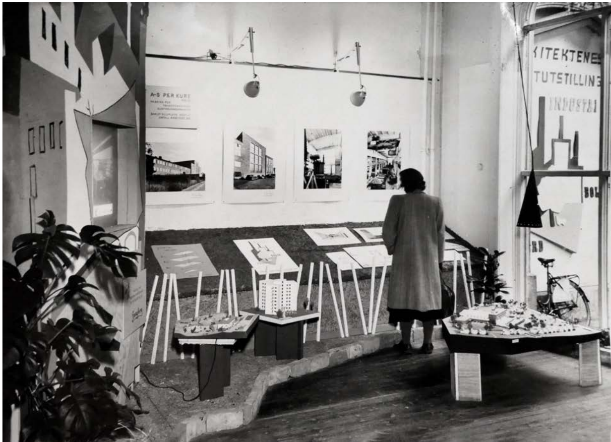
Figure 28 Photograph from the 1949 exhibition on display in Håndverkeren , Oslo. Fagsaker, Norske Arkitekters Landsforbund Archives, The National Archives of Norway, Oslo.
