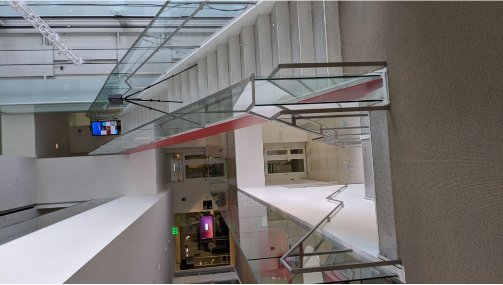
Figure 5-8: We must ensure continuity between floors, so we have to scan every few steps in a staircase.
