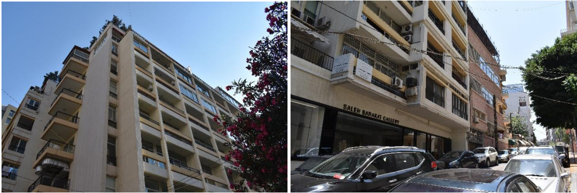
Fig. 38-39. Images of the Building Housing Saleh Barakat Gallery. Images taken by the author.
