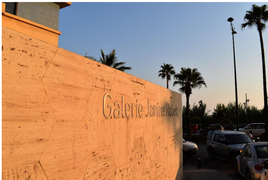
Fig.32. Hexagonal Travertine Exterior Cladding of Galerie Janine Rubeiz. Image taken by the author.
