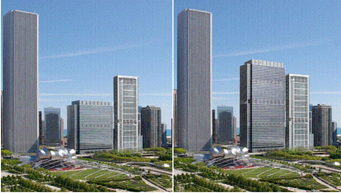
Figure 4-12: Health Care Service Corporation (HCSC) headquarters in the center of image before and after vertical phasing (adapted from [117]).
