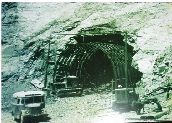
Early construction operations
