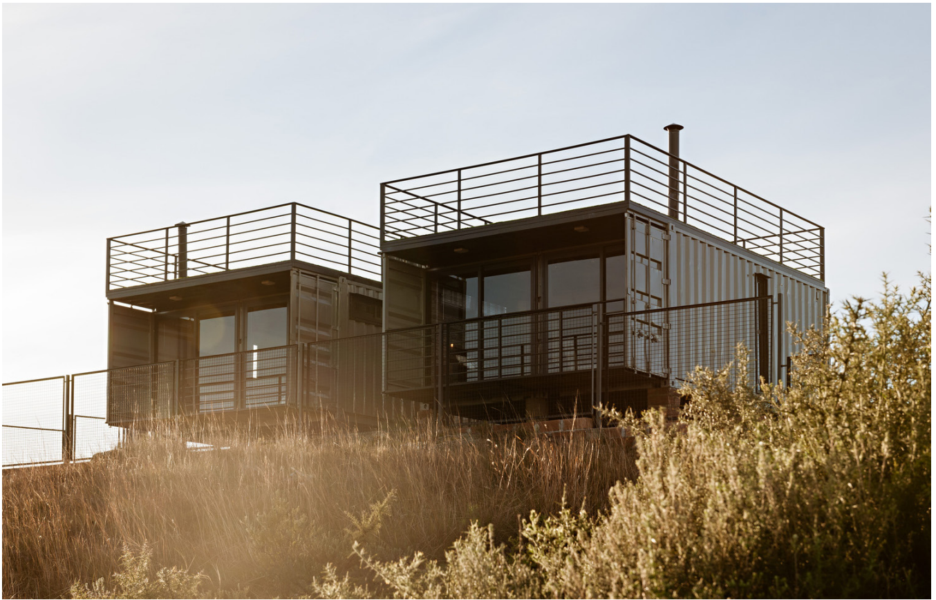
Fig. 24: Cambara Container House (Jordani, 2020)
