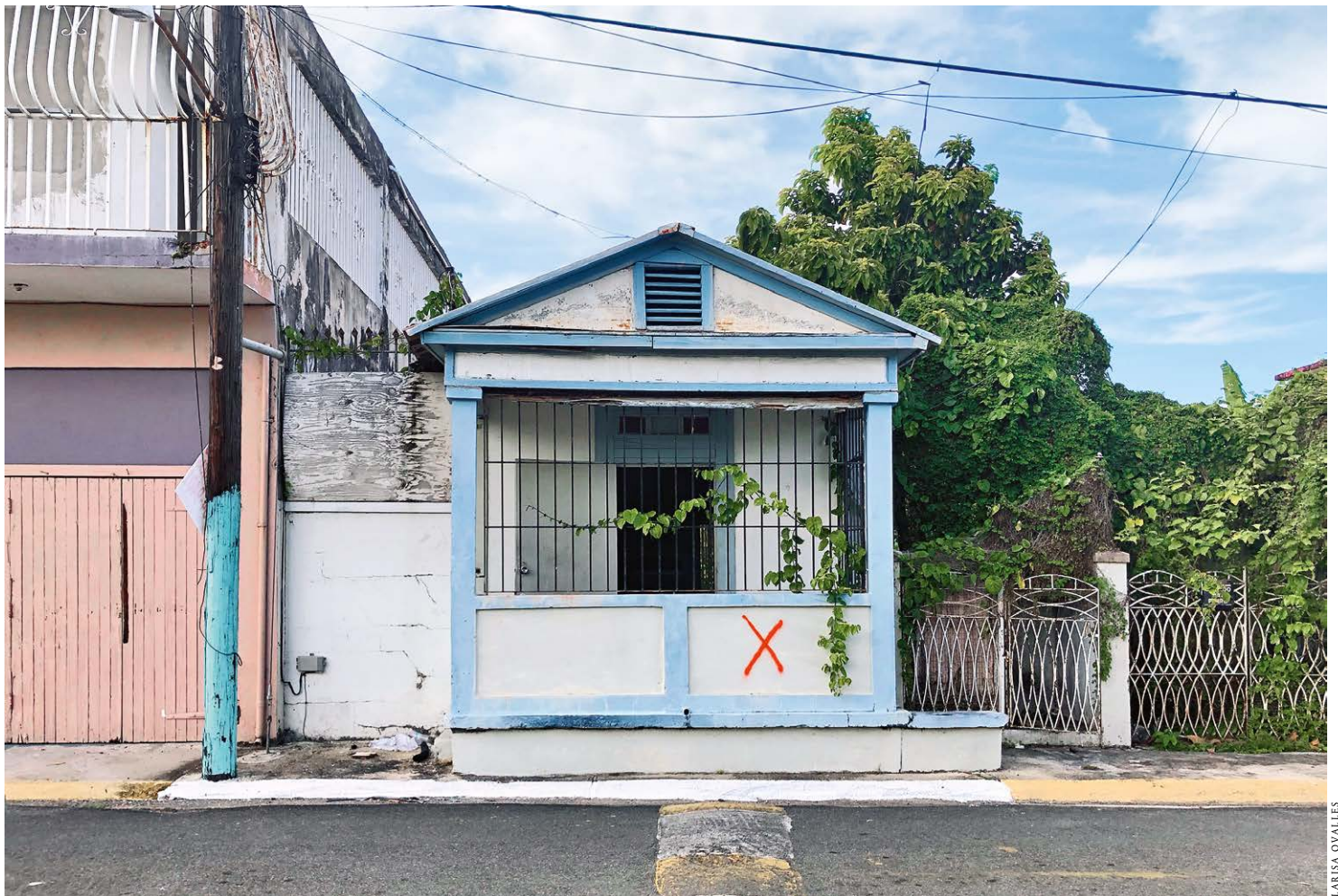
Figure 1 Home marked for demolition post-Maria in Catano, Puerto Rico, March 2019. It is estimated that 49 per cent of Puerto Ricans live in landslide hazard zones. More than 200,000 homes are located in flood zones, of which certain communities are being targeted for relocation. 9
