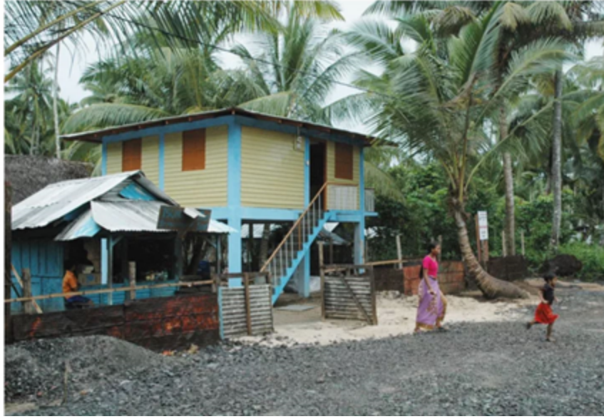
Figure 2: “Prototype tsunami-resistant shelter in Car Nicobar in the Bay of Bengal, India. Photo by Pallava Bagla/ Corbis Historical/ Getty Images. Features the 2 nd level safe rooms for better tsunami and flood resistance. (Craven, 2019).
