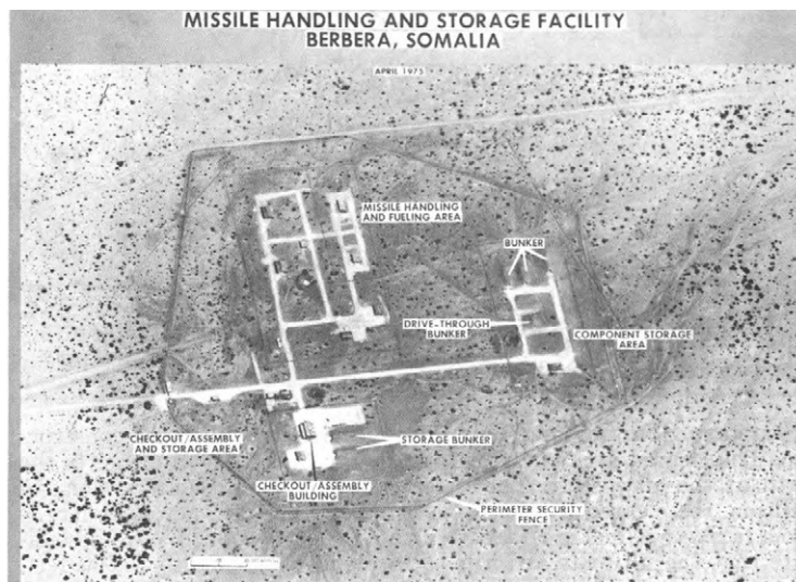
Figure 10. The missile handling and storage facility, a fenced, secured area in Berbera, Somalia. 34
