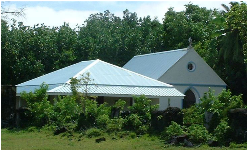
Figure 60. The refurbished chapel at East Point (2002). Source: Ted A. Morris, Jr.
