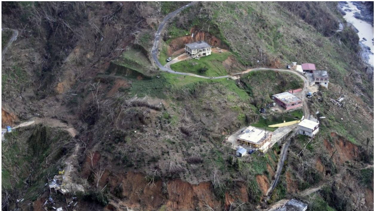
Figure 5-1. Damaged homes near a washed-out road in Utuado, Puerto Rico, on October 3, 2017 (Photo: Eric D. Woodall/US Coast Guard/AP).
