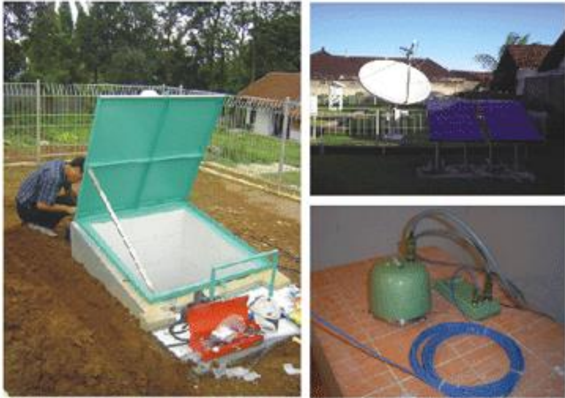
Figure 3-7: A typical seismic station operated by BMKG [26]
