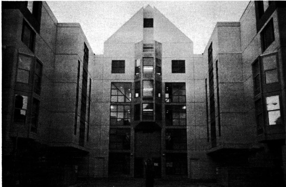
Fillmore Center: development entrance along Eddy Street
