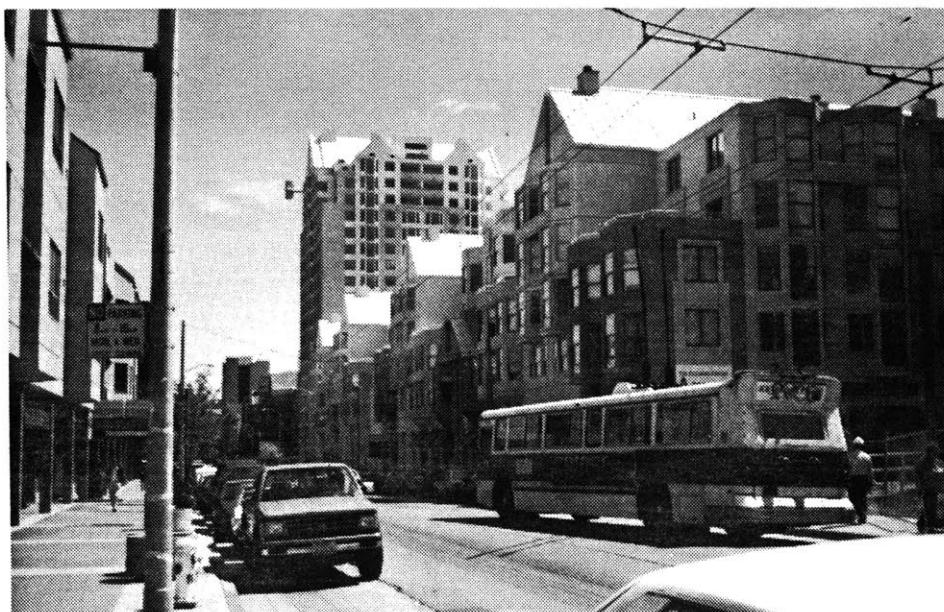
Fillmore Center: Looking south along Fillmore Street
