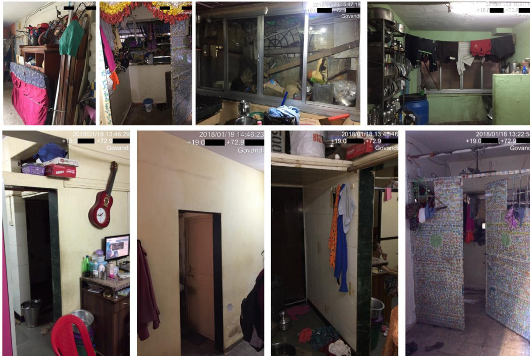
Figure 5. Top row: permanent window obstructions observed in resettlement dwellings inhibiting ventilation paths and natural light. Bottom row: Units retrofitted with low-cost partition walls by occupants.
