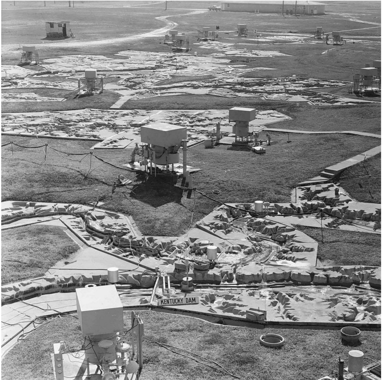
/ Partial Overview of the Mississippi River Basin Model / Eugene Reybold, in operation from 1949-1973 US Army Corps of Engineers
