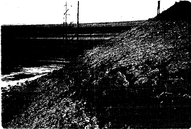
a) Initial toe bulge May 1965
