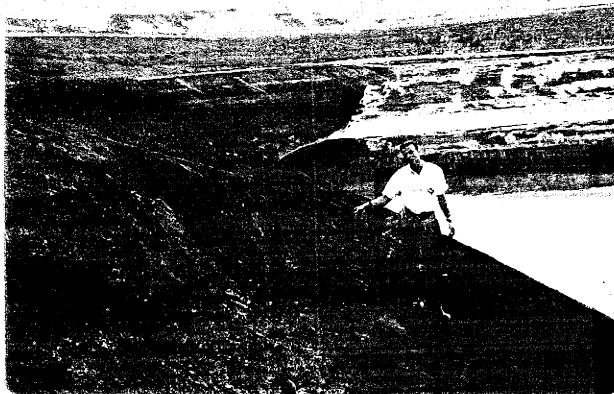
b) Development of wedges during the slide May 1965
