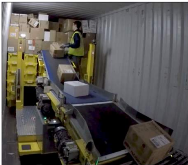
Figure 4-4: Powered-tilt conveyor for trailer unloading
