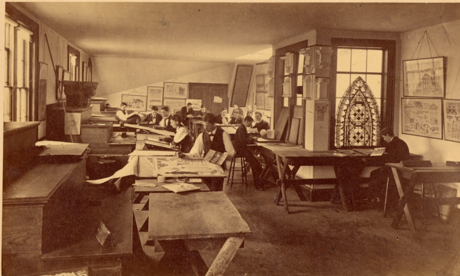
FIFTH FLOOR DRAFTING ROOM IN 1876 DRAFTING ROOM IN 1929
