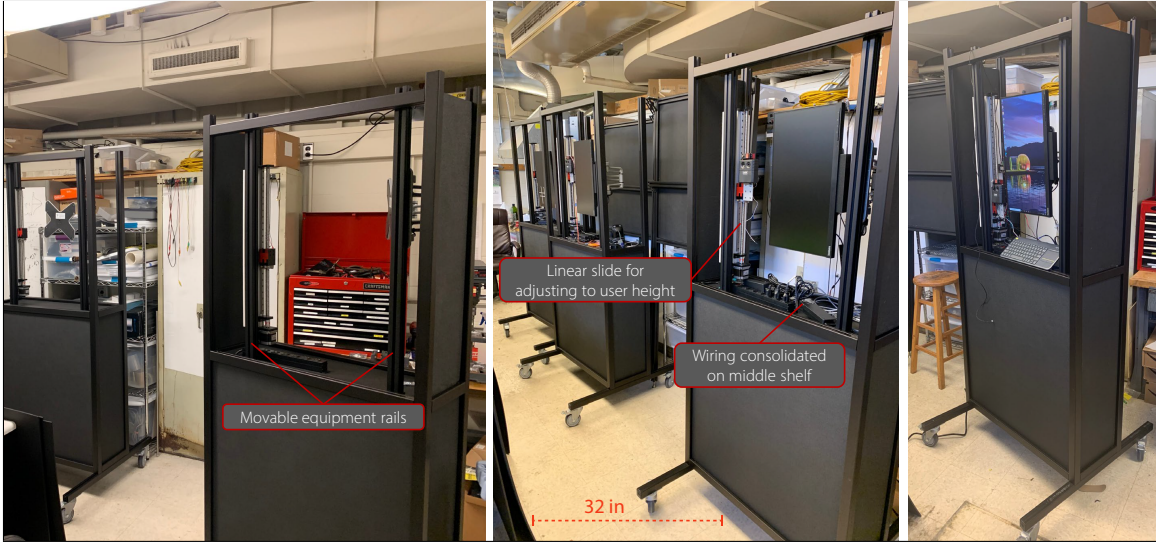
Figure 2-4: Frame assembly process.
