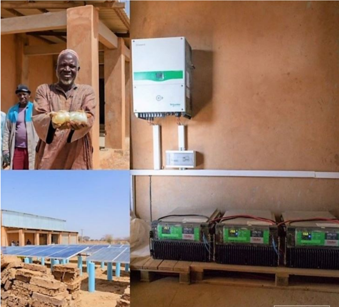
Figure 3-5: FZSONICK batteries installed in Senegal to store energy from a solar farm to refrigerate a granary. Source:(FZSONICK, 2021). Reproduced with permission of the copyright owner.
