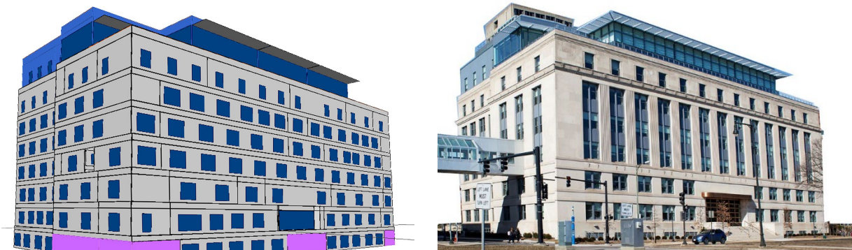
Figure 4-11: Left, rendering of the developed energy model; Right, a photograph of the building post-renovation.
