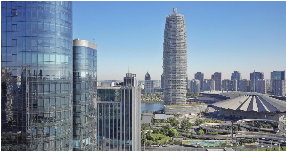
Figure 13. Towers in the CBD Area Source: Administrative Committee of Zhengdong New District
