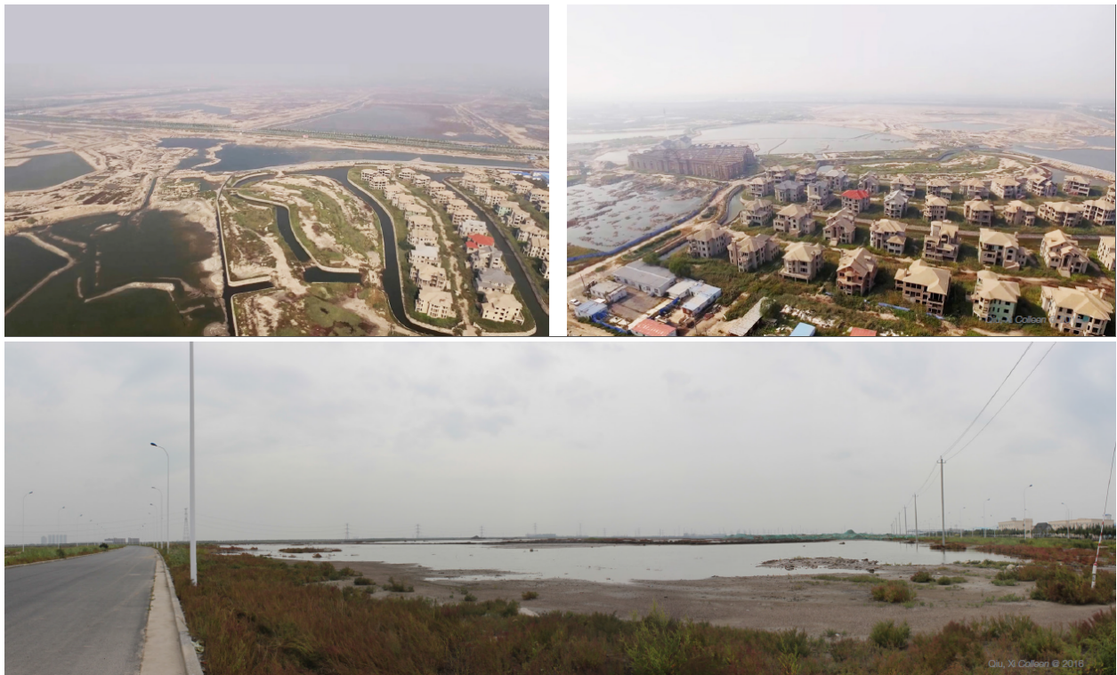
Figure 10. Parts of the Tianjin Eco-City in 2017 (photos by author)
