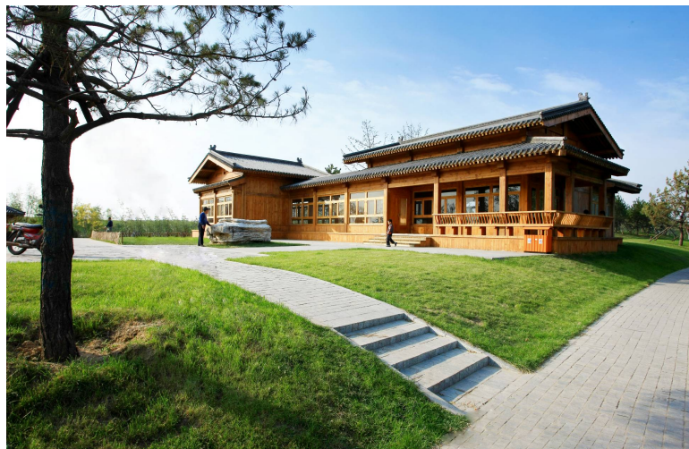
Figure 26. “Light timber framed buildings were built in consideration of limited ground bearing capability, traditional Chinese culture, resource and energy consumption, and environmental effects on the park.” Source: Tsinghua Tongheng Planning and Design Institute
