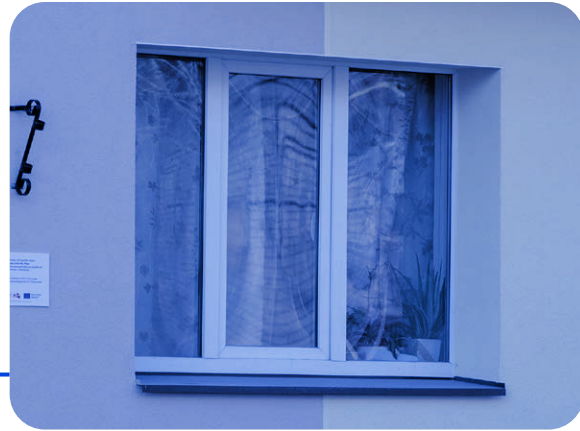
New double pane windows
