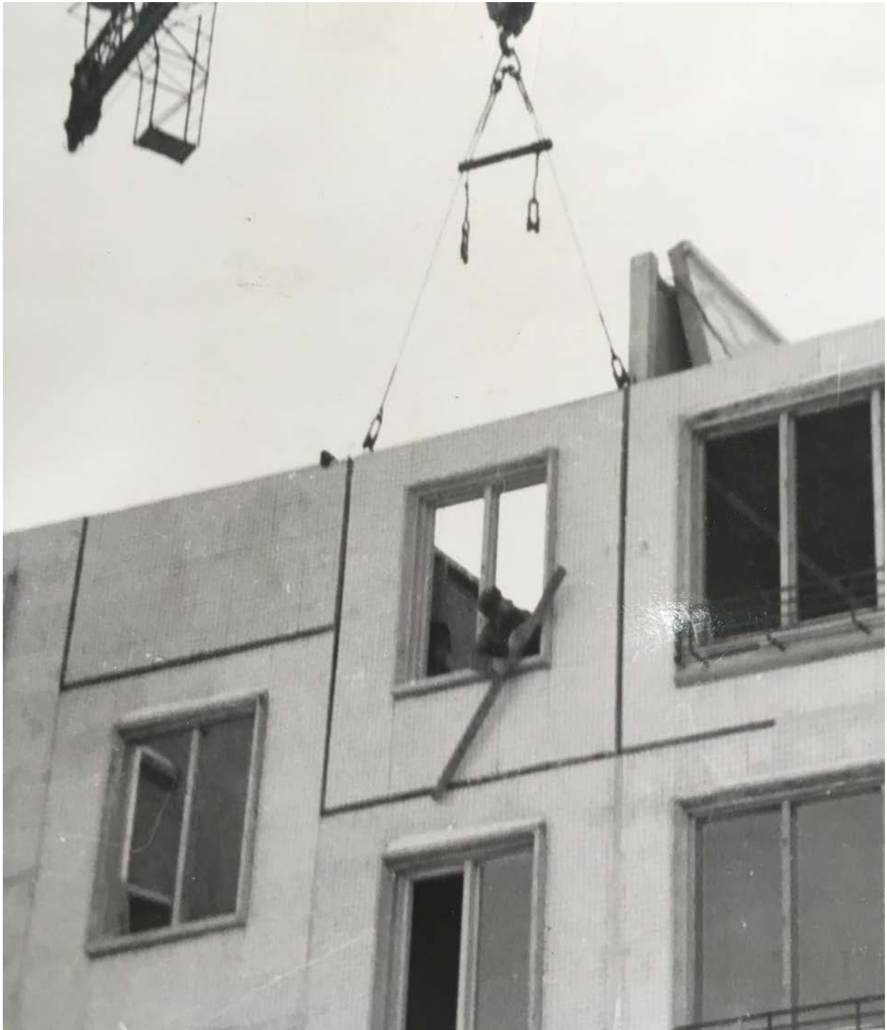
Panel assembly. Source: Photo Archives, Shchusev State Museum of Architecture. Moscow, 2019
