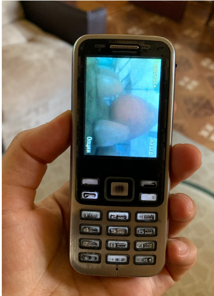
Photo of a photo from the reconstruction of Tatev Monastery, where large ceramic vessels are buried inside the mortar to reduce the weight of the dome, conserve on mortar, and produce an echoing effect under the dome.
