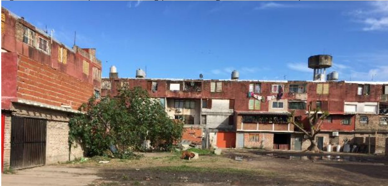
Figure 38. Vertical expansions showing partial blockages of second floor apartments' windows
