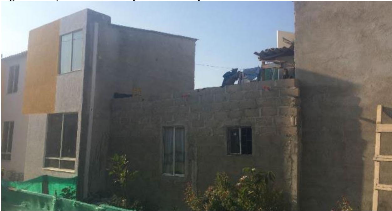
Figure 85. Expansion at the backyard of two-story house
