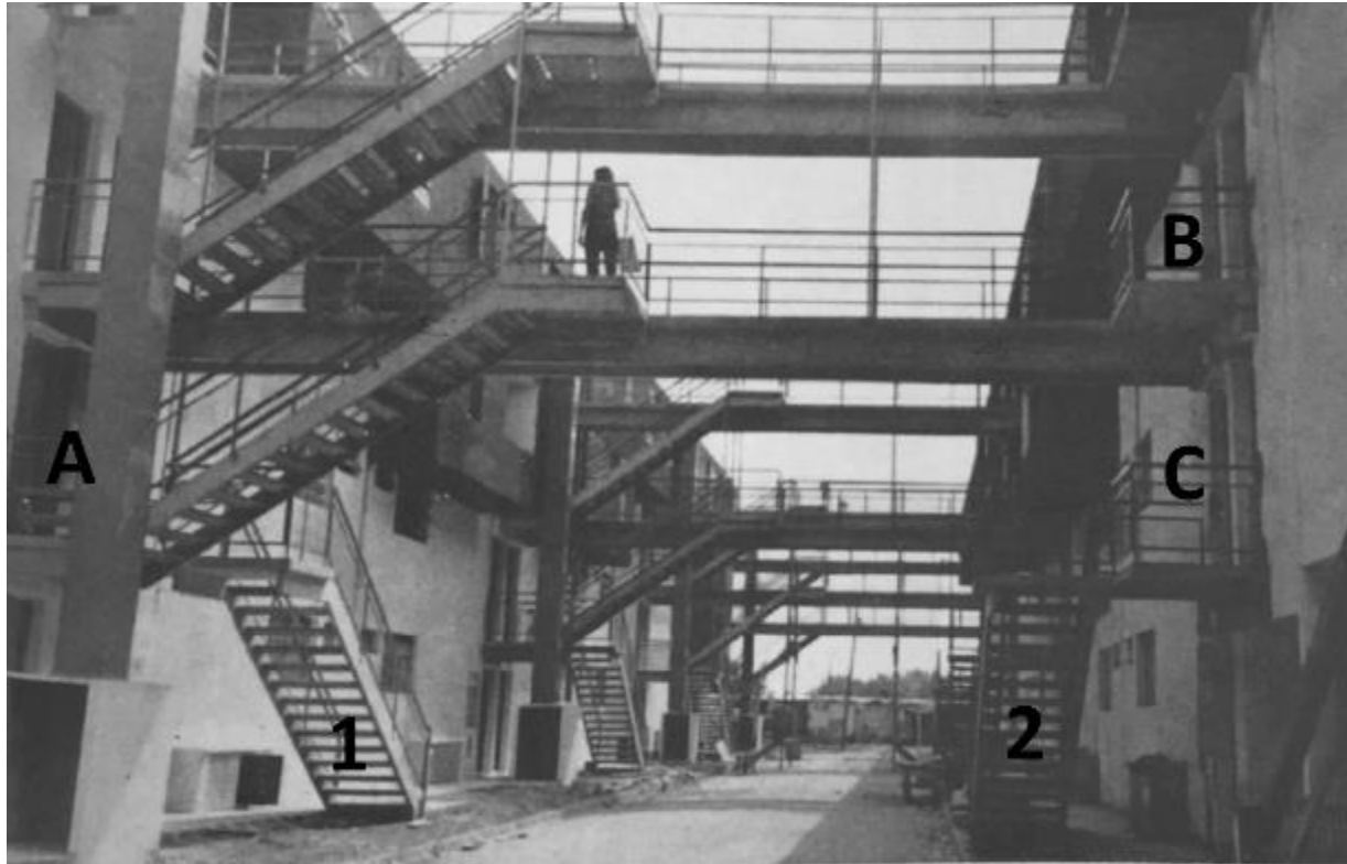
Figure 14. Staircases and bridges
