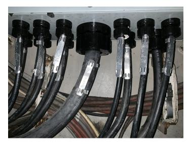
Figure A-18: Cables entries into the bottom of 1S-4P-(2-32-1).
