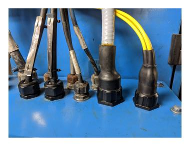
Figure A-16: Example of voltage leads (in conduit) and Conxall cables exiting from power panel.
