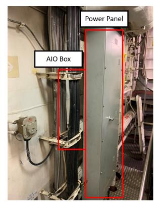
Figure A-7: Proposed installation location for AIO box on Power Panel 1S-4P-(2-32-1) located in the Engine Room.
