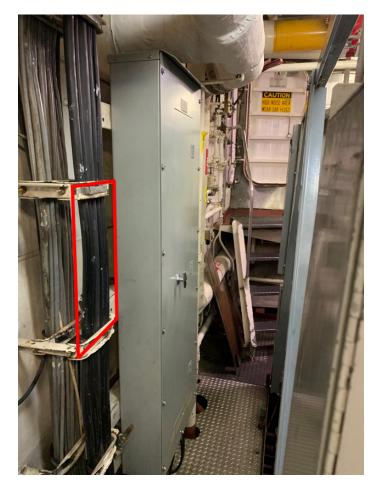
Figure A-9: Proposed mounting location for AIO box in the Engine Room.
