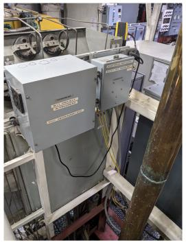
(b) NILM installed on power panel 3-117-1.
