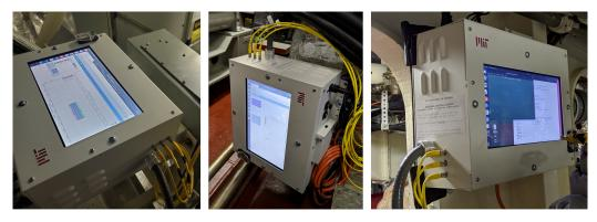
Figure 1-5: Installation of three NILMs on USS INDIANAPOLIS.
