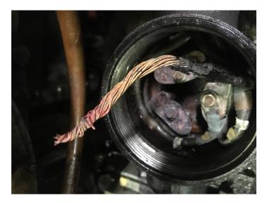
Figure 3-40: Visible corrosion on #1 jacket water heater wiring.
