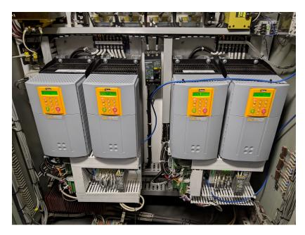
Figure 3-37: Sample of exciters located within the main switchboard cabinet.
