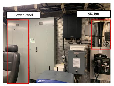
Figure A-6: Proposed installation location for AIO box on Power Panel 1S-4P-(1-66-2) located in the Engineering Control Center (1-58-0-C).
