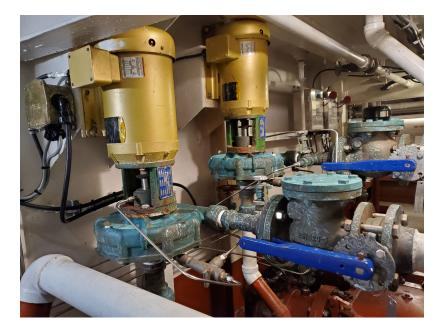
Figure 3-34: Main motor cooling pumps.
