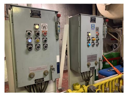
Figure 3-29: USCGC THUNDER BAY Engine Room Supply Fan Controllers
