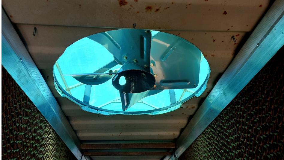
FIGURE A-2: Pad Support and Fan Installation in Full-Scale
