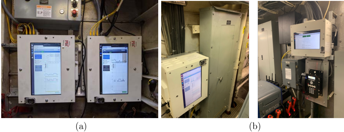
Figure A-7: NILM installations on (a) USCGC Marlin and (b) USCGC Thunder Bay.
