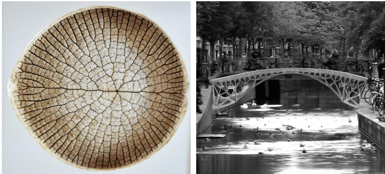
Figure 03 Laarman 3D Printed Bridge through Biomimicry: Amazon water lily structure - Reprinted from pangaeaproject.com, 2013 (Left). Elevation of 3D printed bridge mimicking the branching strategy for the bridge's structure - Reprinted from dezeen.com, 2021 (Right).
