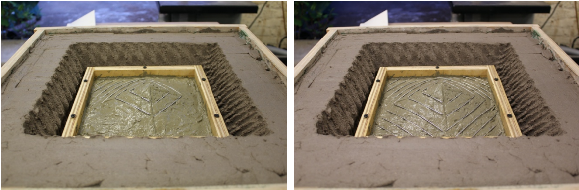
Figure 36: Adding rebar to thin concrete shell on adobe formwork
