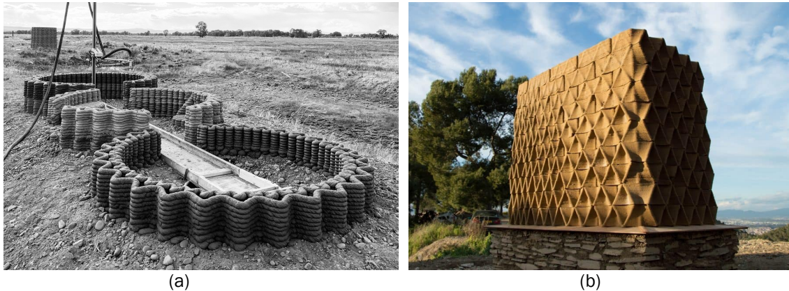
Figure 11: Full scale 3D printed earthen wall structures by (a) Curth et al. (image courtesy of Curth), and (b) Dubor et al. (IAAC)
