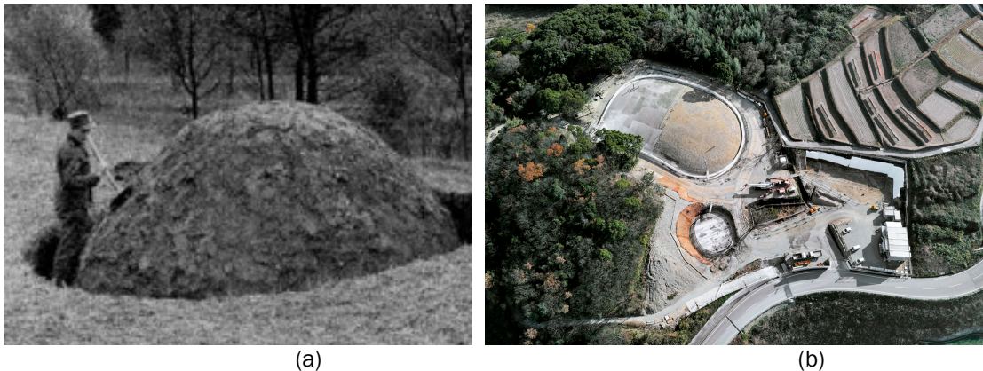
Figure 10: (a) Isler's freely shaped hill method (Gericke et al. 2016), (b) Earth formwork for the Teshima Art Museum (ArquitecturaViva)
