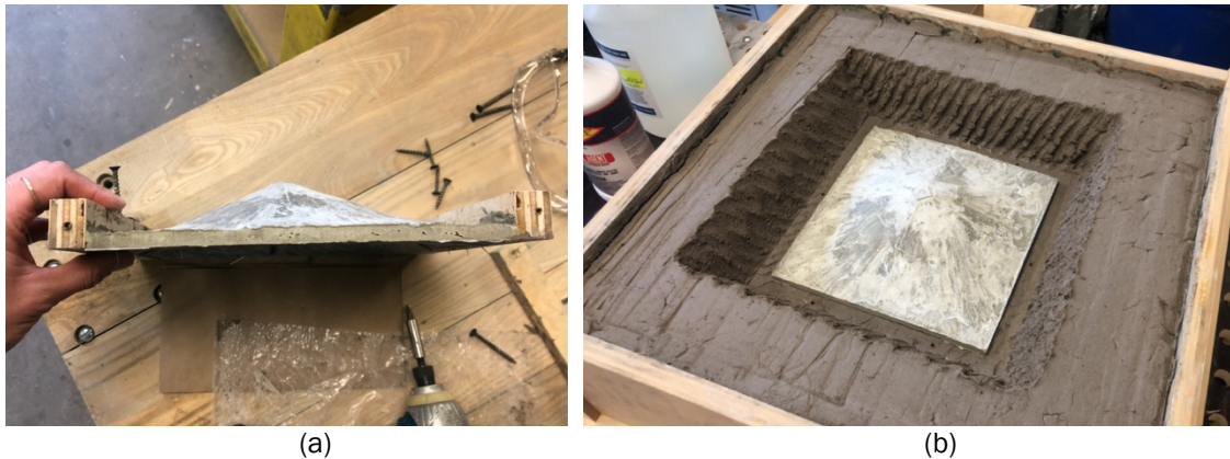
Figure 38: (a) Side view of cured concrete shell foundation, and (b) cured concrete shell on adobe formwork
